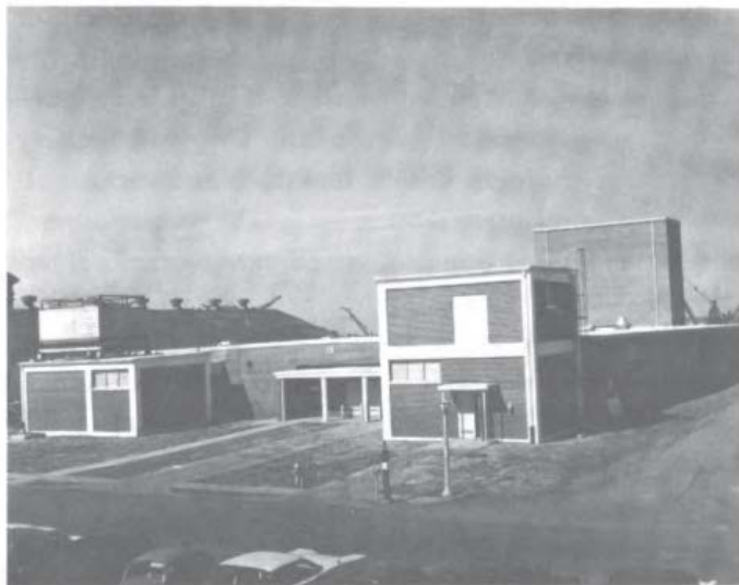
Figure 1. New facility provides special environmental conditions, including temperature, humidity, dust and vibration control required for precision electronics and optical equipment repairs.
