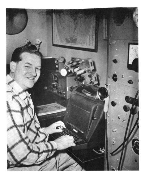
Am enclosing a photo of the station showing the model 26 with mechanical carriage release added. The terminal unit is 6AEE with some minor variations. Receiver in upper right is a variable tuned 522 and 522 companion transmitter at bottom. Antenna is a ground plane. Oper-
