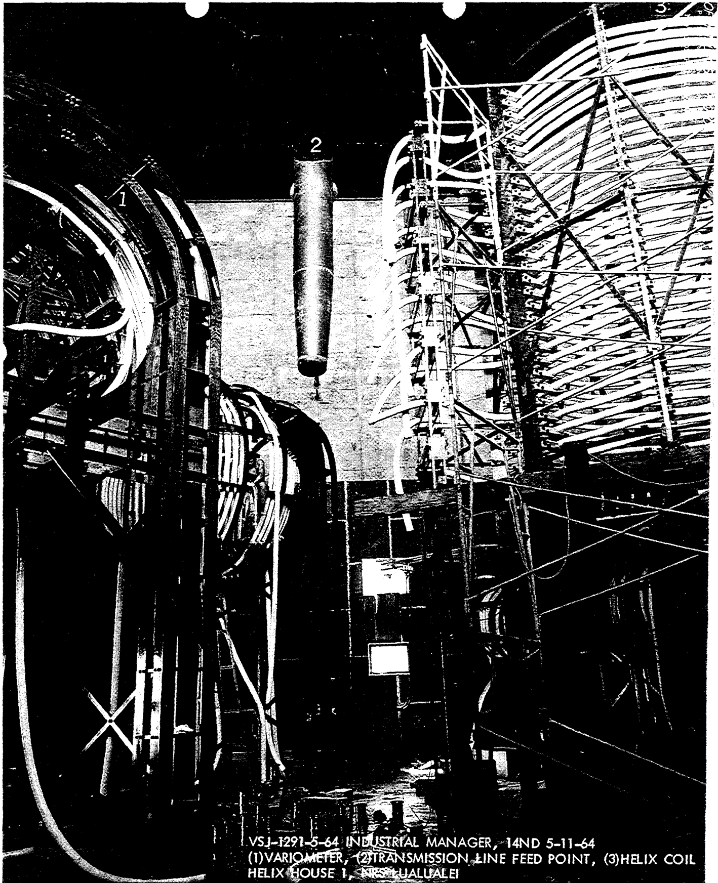
Figure 15. Photograph No. VSJ-1291-5-64 - "(1) Variometer, (2) Transmission Line Feed Point, (3) Helix Coil, Helix House 1, NRS Lualualei," dated 5/11/55 (RTF-Lualualei Collection).
