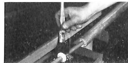
*Cleaning the inner conductor of a coaxial transmission line.*
