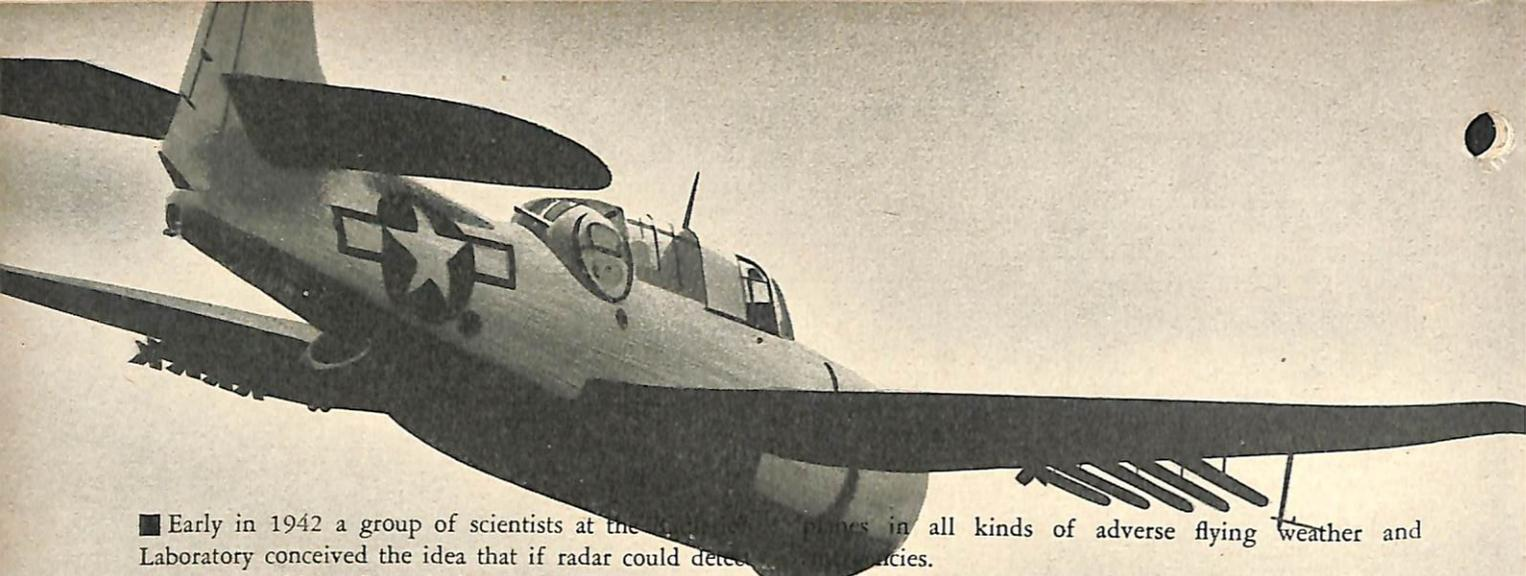
Early in 1942 a group of scientists at the Naval Research Laboratory conceived the idea that if radar could detect the exact position of an airplane at any given moment, this information could be used to guide the airplane to a safe landing through fog, darkness, or other conditions which previously had made landings impossible or extremely hazardous. This idea came to be known as GCA (Ground-Controlled Approach).
