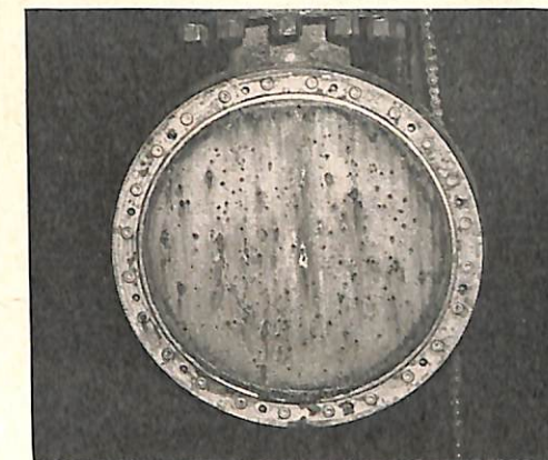
Projector face before cleaning, showing pitting and sea growth.
