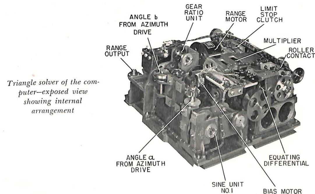
Triangle solver of the computer—exposed view showing internal arrangement
