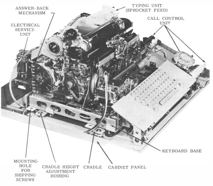
Figure 5 - 35 KSR Set With Cover Removed
