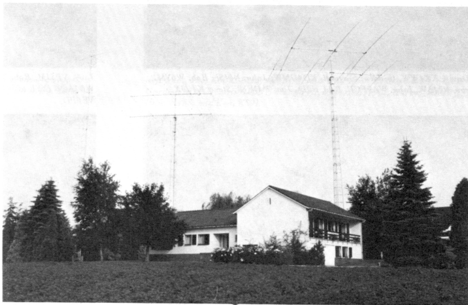
Antennas at ON4UN, 10 mtr: 6 El. at 60ft., 15 mtr: 6 El. at 70ft., 20 mtr: 5 El. at 85ft., 40 mtr: 3 El. at 100ft., 80 mtr: 85ft. vertical and 135ft. vertical, 160 mtr: 135 ft. vertical and beverages (1000ft. long in 12 directions)
